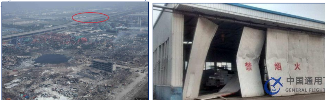
Figure 11 - Location of Binhai airport, where four helicopters sustained unknown levels of damage by the shock wave and the hangar door buckling (Images: Panorama/Google, General Flight of China)
