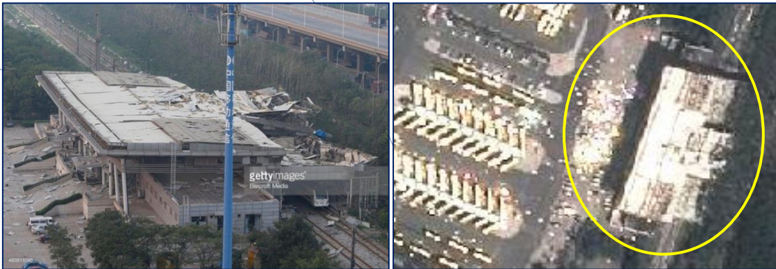
Figure 10 - Donghai Road light rail station, which sustained severe damage in the blast (Images: Getty, Airbus Defense & Space):
